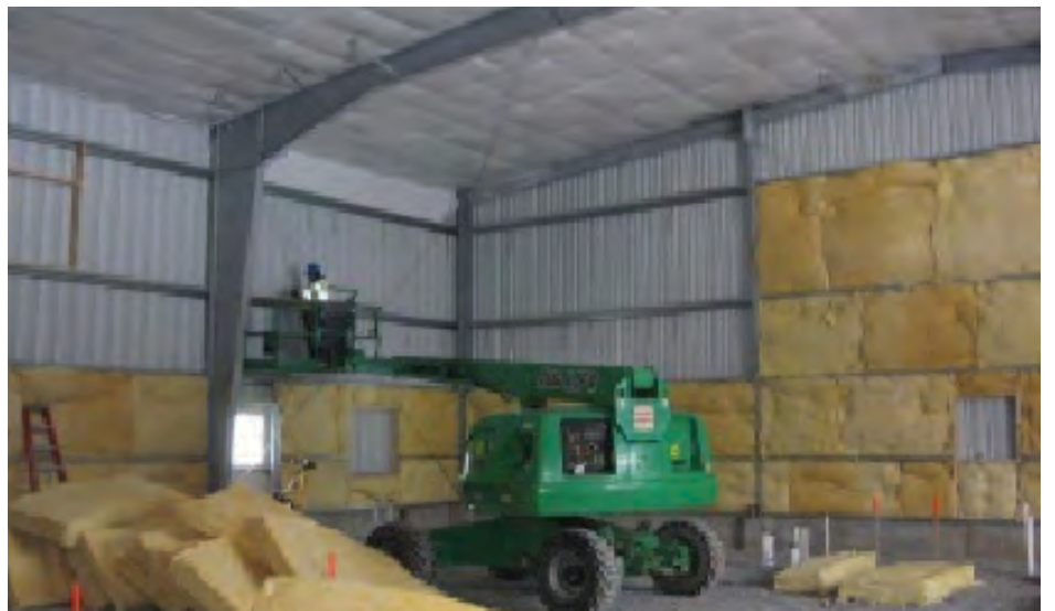
The energy-efficient building is insulated as inside finish work began.
