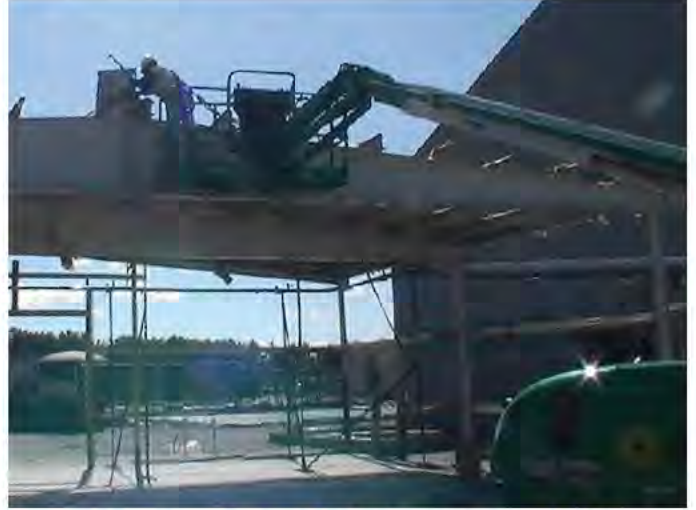
A warm winter day and a hot cutting torch help a worker as the final structure of a site building is taken down.
