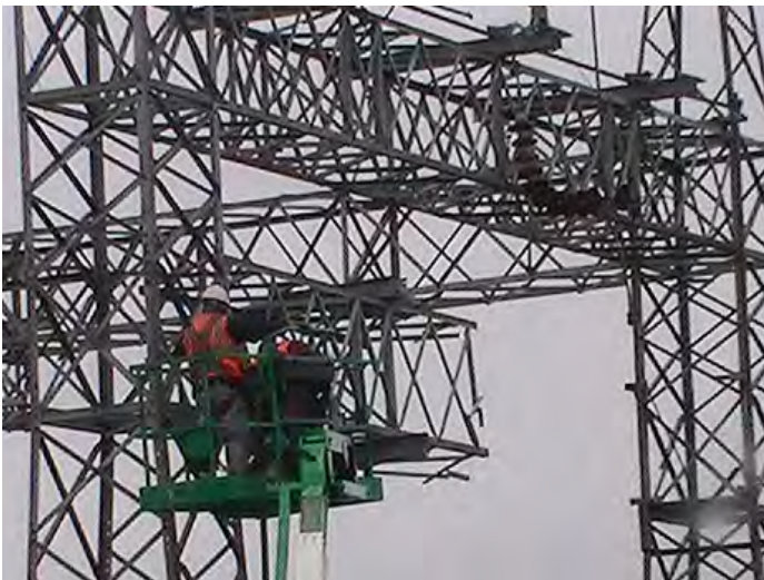
Workers remove the maze of steel that once held the plant's power transformer.
