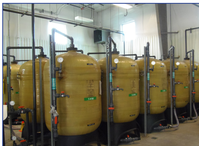
These tanks contain Mersorb and Granulated Activated Carbon which remove mercury and other contaminants from extracted groundwater before it is discharged in compliance with the MEPDES Permit.
