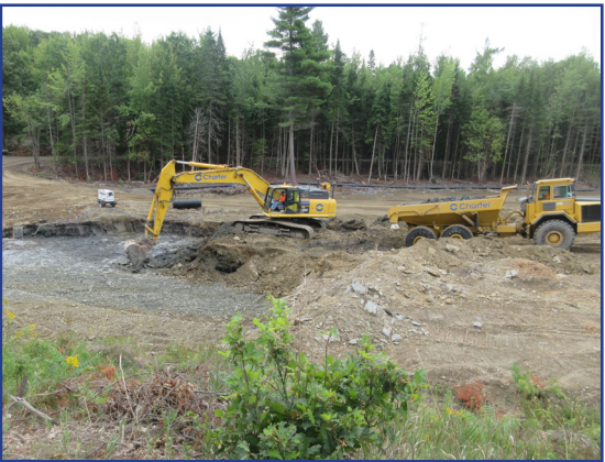
One of the big numbers driving the remediation is the amount soil excavated and hauled off site for safe disposal. The cycle begins with extensive soil and water analysis and then moves on to excavation, disposal, back filling with new soil and then vegetating the area with new grass and plant life. The photos above (top left and clockwise) show that cycle with the Southerly Stream and the Scrap Metal Yard in before and after photos.
