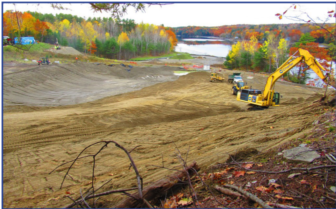
The fall weather was ideal last October as site workers back-filled the area where Landfill 1 was located with clean soil before it was then groomed and readied for new vegation.
